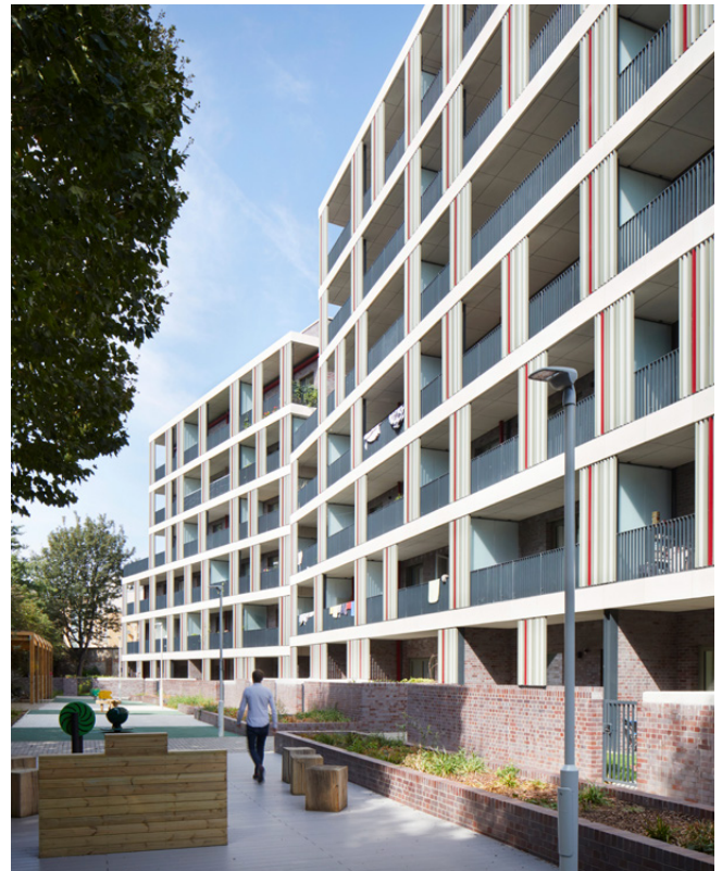
Figure 37 – Illustrative example of urban renewal - Agar Grove, Camden (Credit Jack Hobhouse; Hawkins Brown Architects)
