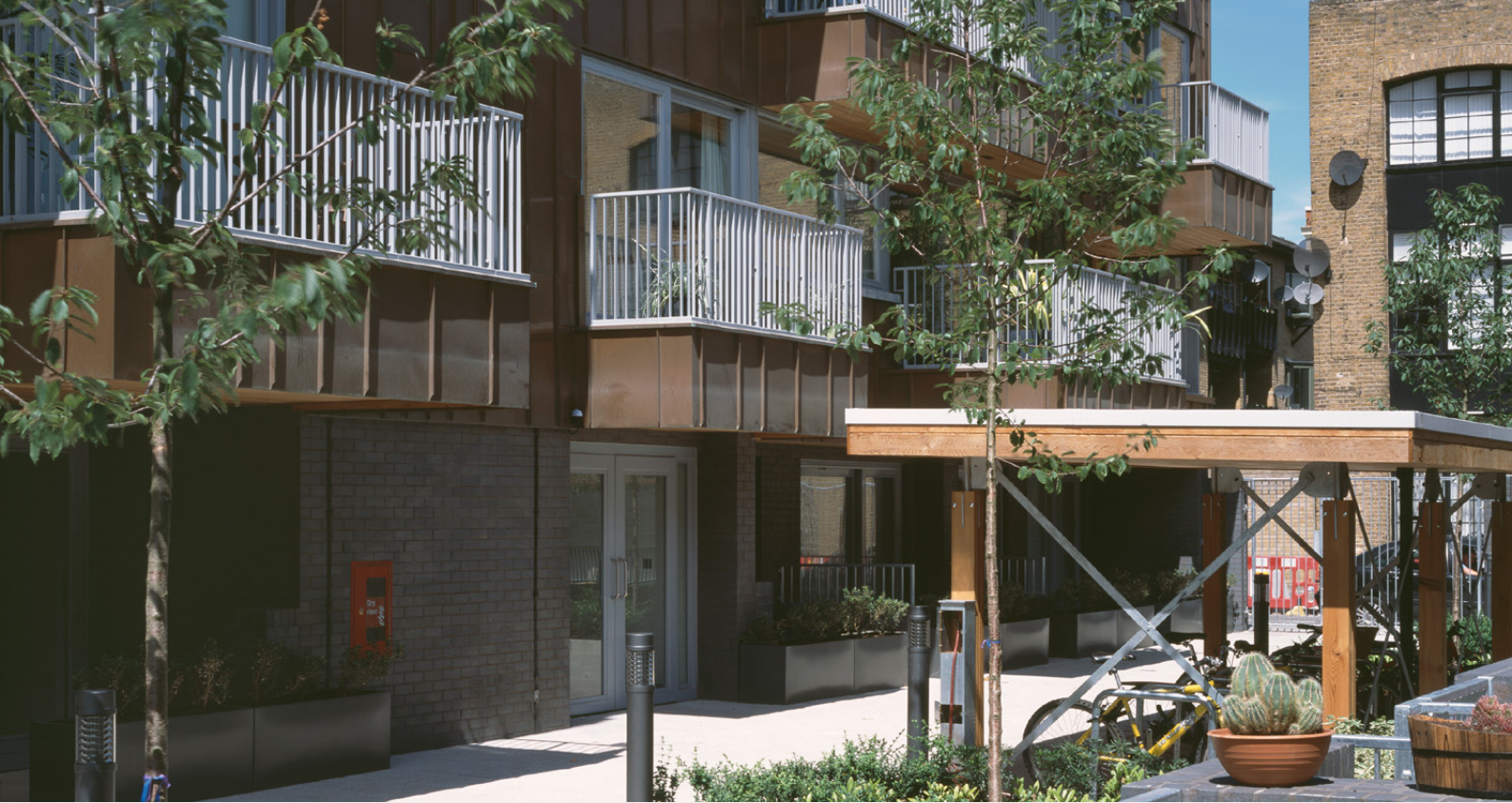
Figure 7 – Illustrative example of urban development at Claredale St, East London (Image credit Ioana Marinescu, Karakusevic Carson Architects)
