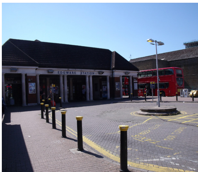
Figure 19 – Edgware Station and forecourt
